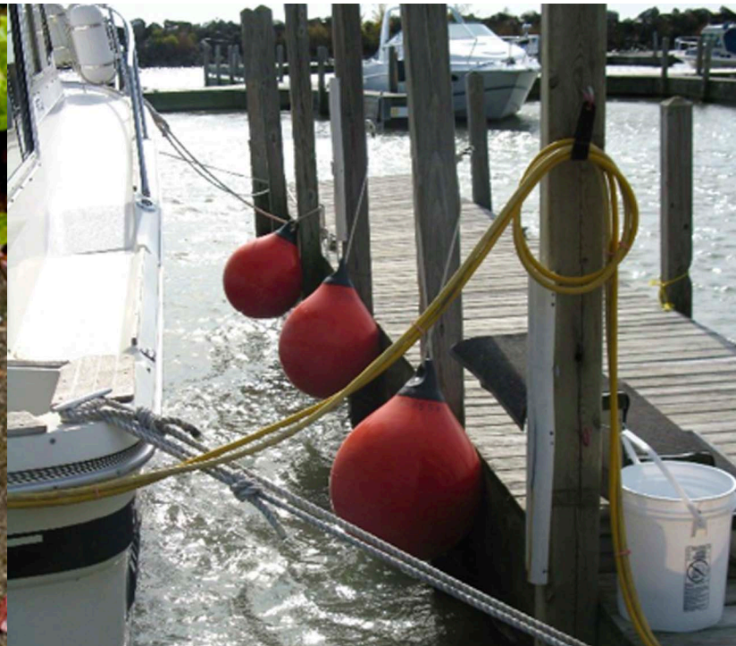
Figure 14: The Colchester Harbour Marina, was the first to have a floating dock in all of the Windsor-Essex region. A floating dock is more suited to adjusting to fluctuating lake levels and storm-prone regions, as opposed to fixed docks that do not adjust to lake levels.
