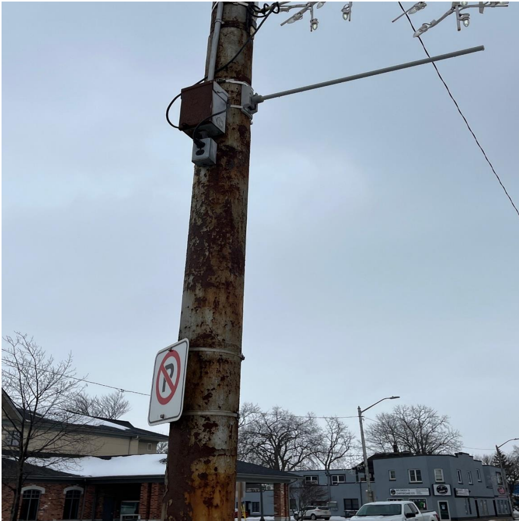
Figure 5: Essex Centre Streetlight Poles
