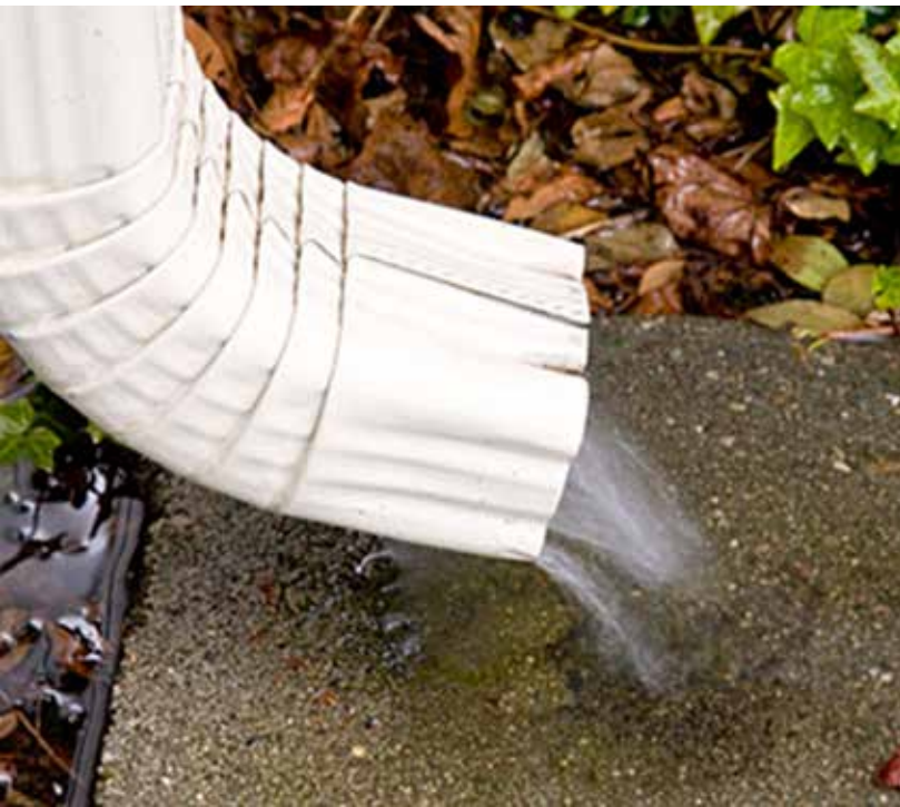
Figure 13: The Town of Essex has implemented its Downspout Disconnection and Basement Flooding Subsidy Programs to assist homeowners in reducing site-level flooding issues caused by increased precipitation in the region.
