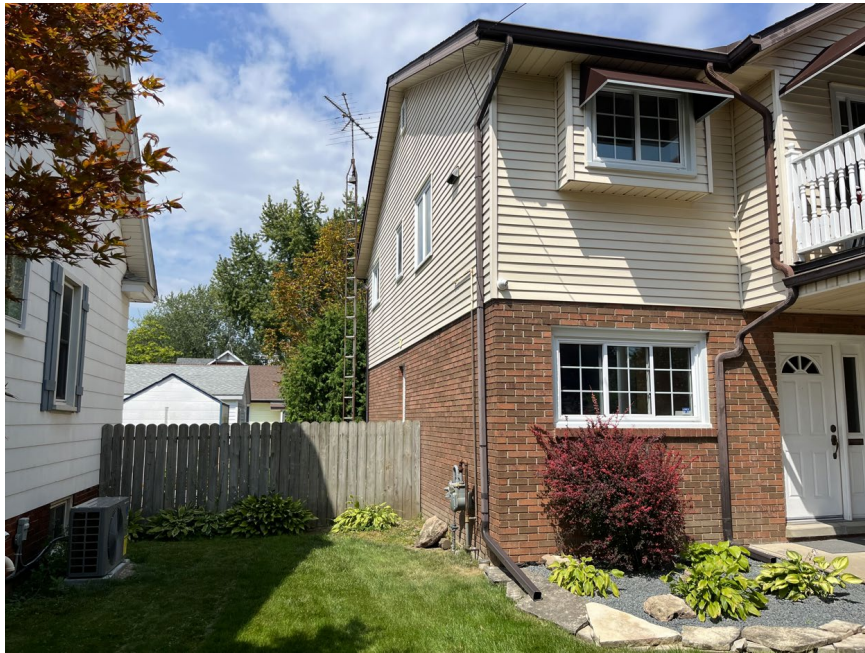
Southern interior side yard
