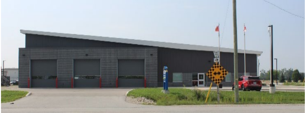
Figure 8. Exterior of Station 2 – Gesto.
