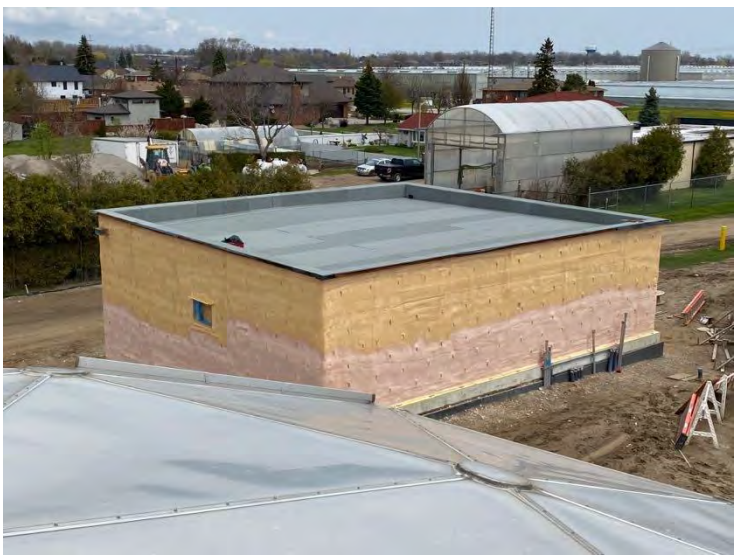
62. Auxiliary Building – Spray Foam (2022-05-05)
