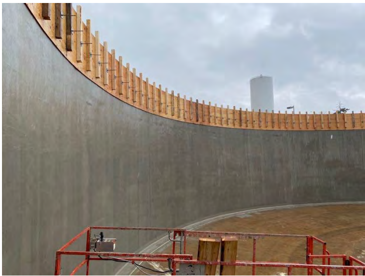
33. DAF No. 1 Tank – Interior Forms (2022-05-03)
