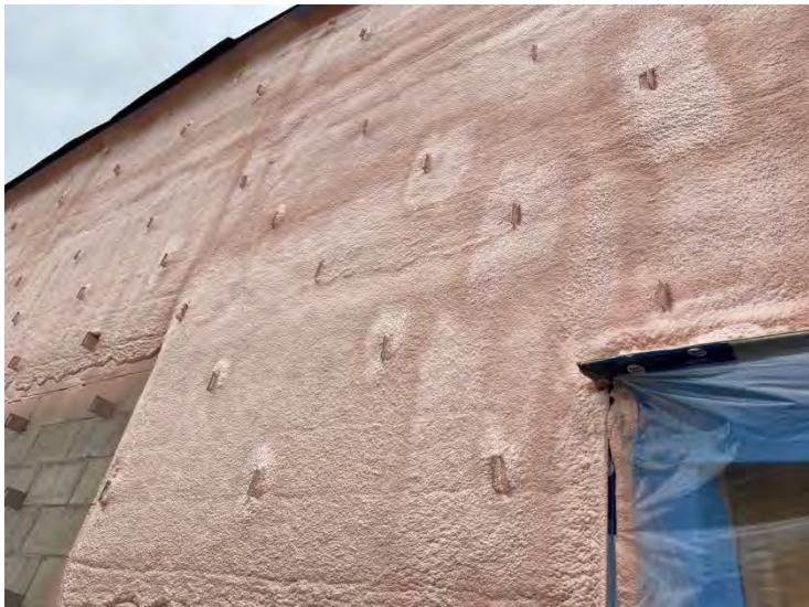
16. Auxiliary Building – Spray Foam Insulation (2022-05-02)
