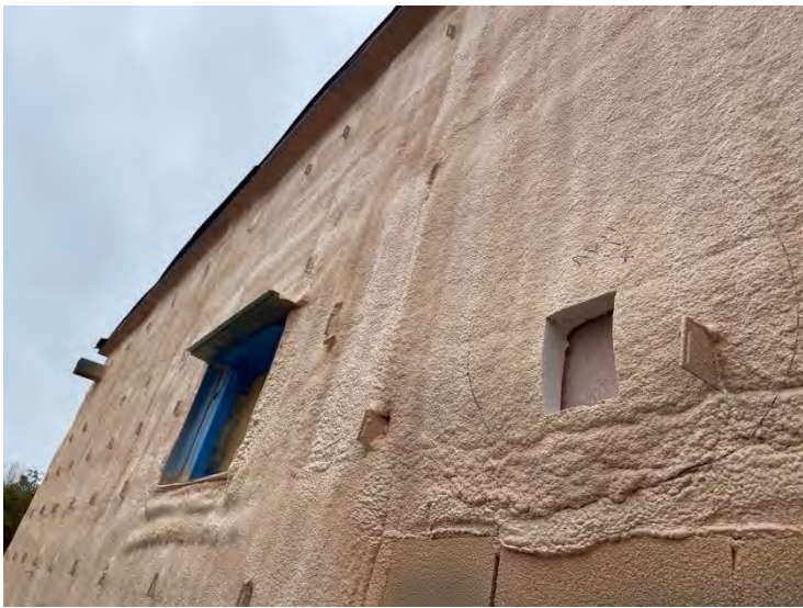
42. Auxiliary Building – Spray Foam Third Party Inspection Hollow Area Marked Out (2022-05-04)
