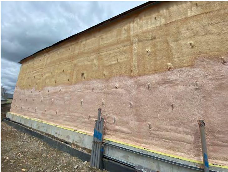
66. Auxiliary Building – Spray Foam (2022-05-05)
