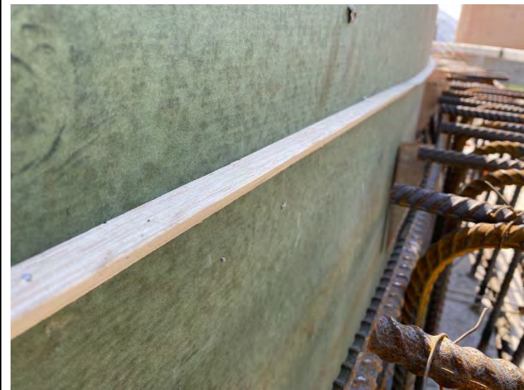
55. DAF No. 1 Tank – Interior Formply Chamfer Strip (2022-05-04)
