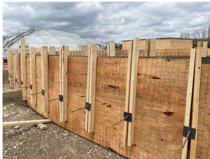
60. DAF No. 1 Tank – Exterior Form (2022-05-05)
