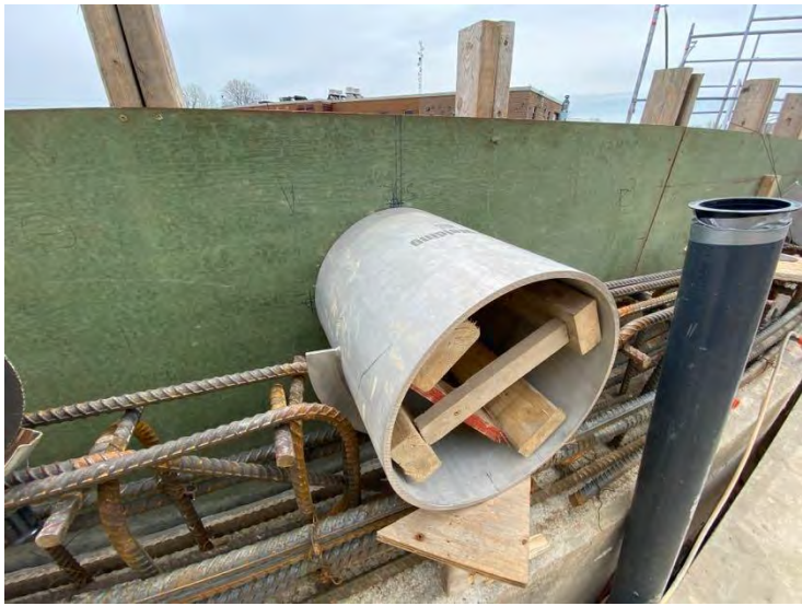
63. DAF No. 1 Tank – Spool with Partial Flange for Saturation Pipe (2022-05-05)
