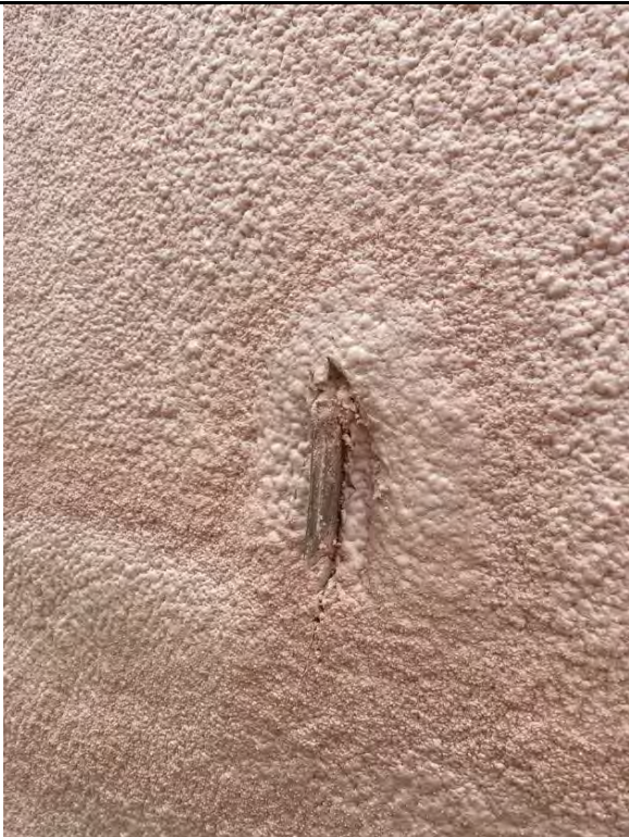
69. Auxiliary Building – Spray Foam at Block Connector (2022-05-05)
