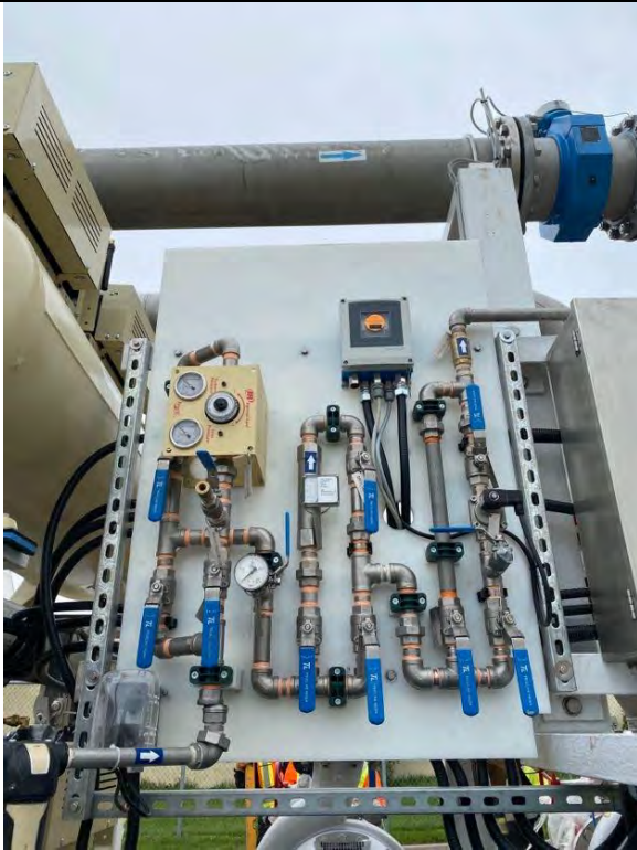
49. DAF No. 1 Saturation Skid (2022-05-04)
