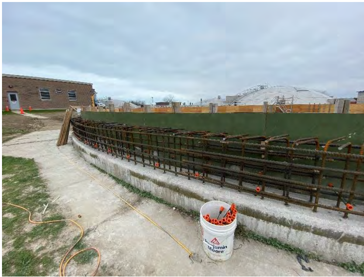
9. DAF No. 1 Tank – Interior Form (2022-05-02)
