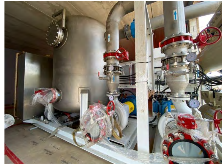
48. DAF No. 1 Saturation Skid (2022-05-04)
