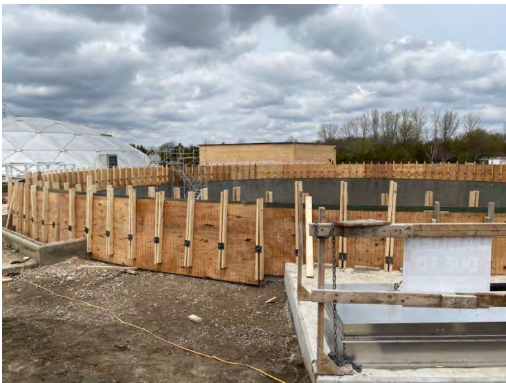
59. DAF No. 1 Tank – Exterior Form (2022-05-05)
