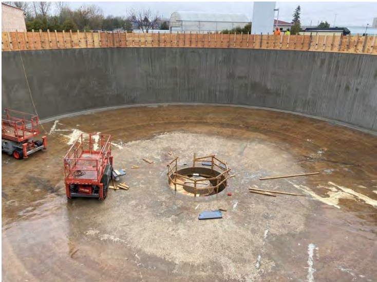
28. DAF No. 1 Tank – Interior Forms and Supports (2022-05-03)
