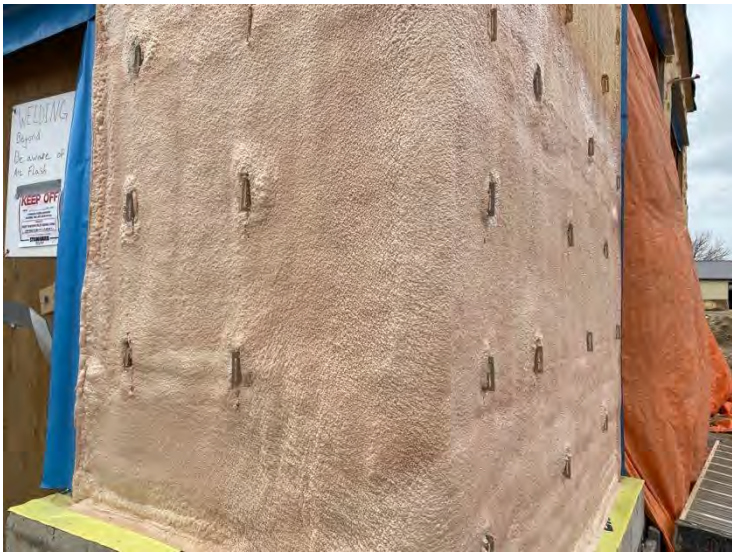
68. Auxiliary Building – Spray Foam (2022-05-05)
