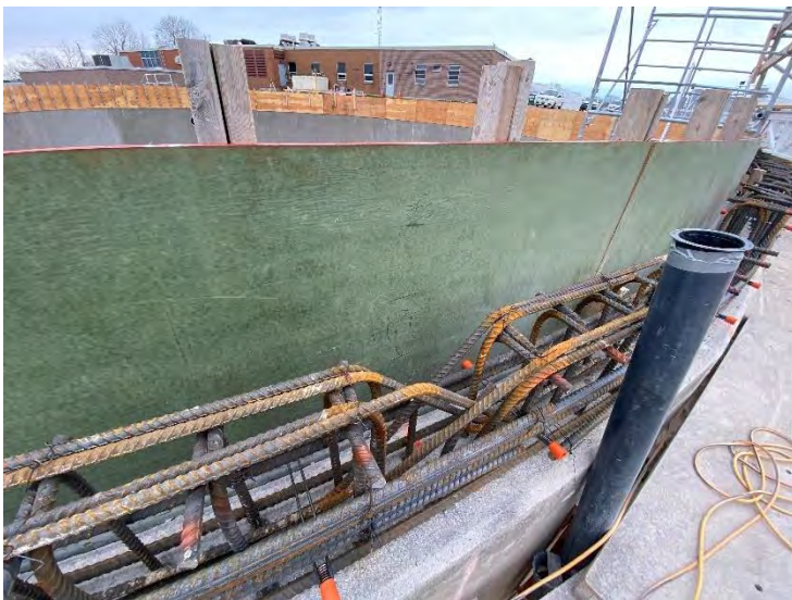
11. DAF No. 1 Tank – Saturation Pipe Reinforcement (2022-05-02)
