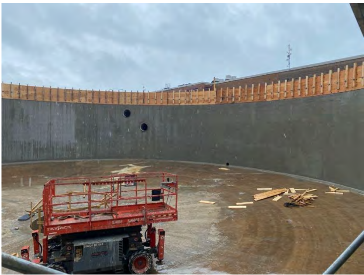
34. DAF No. 1 Tank – Interior Forms (2022-05-03)
