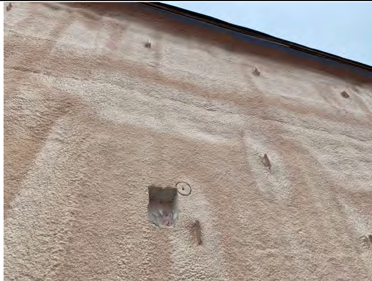
45. Auxiliary Building – Spray Foam Third Party Inspection Sampling Area (2022-05-04)
