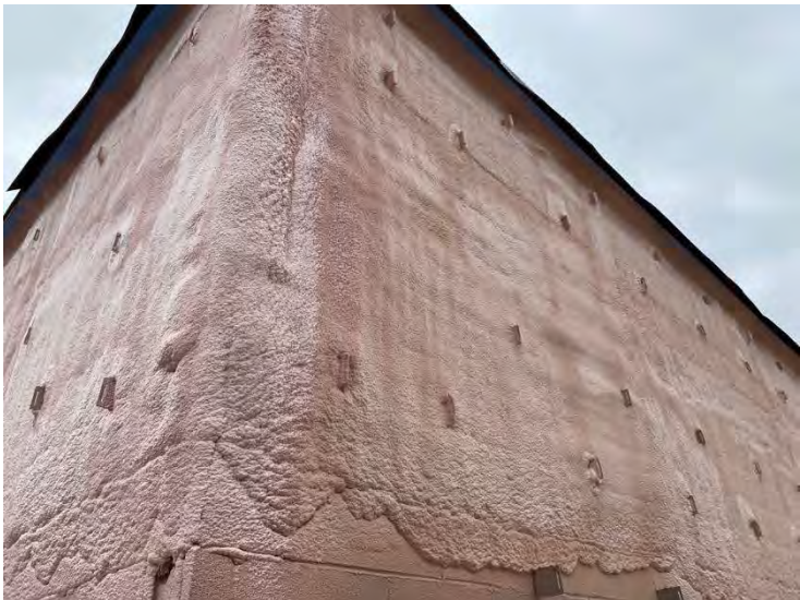
20. Auxiliary Building – Spray Foam Insulation (2022-05-02)
