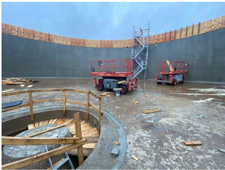
37. DAF No. 1 Tank – Interior Forms on Walls and Centre Cone Form (2022-05-03)
