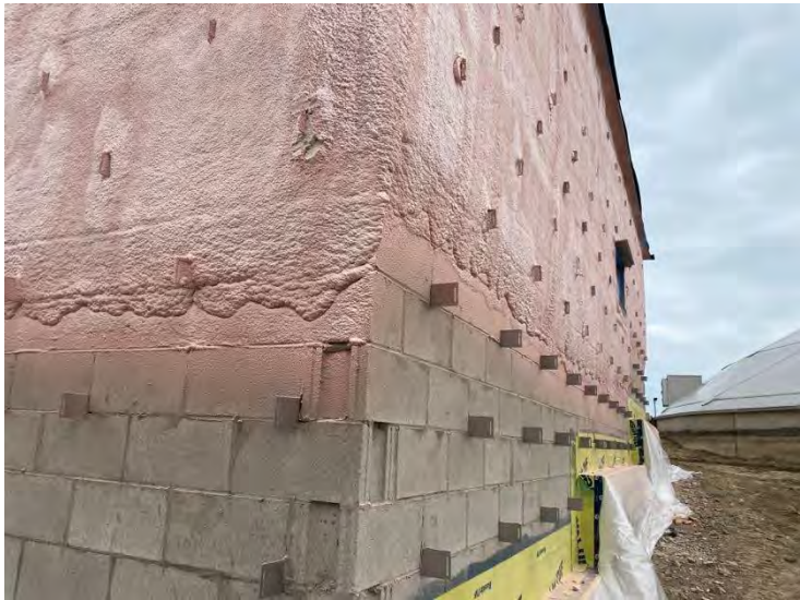
14. Auxiliary Building – Spray Foam Insulation (2022-05-02)
