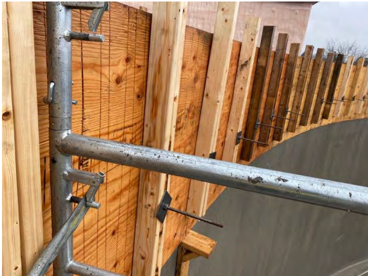
40. DAF No. 1 Tank – Interior Forms (2022-05-03)
