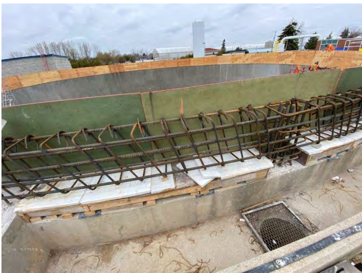
4. DAF No. 1 Tank – Interior Form (2022-05-02)
