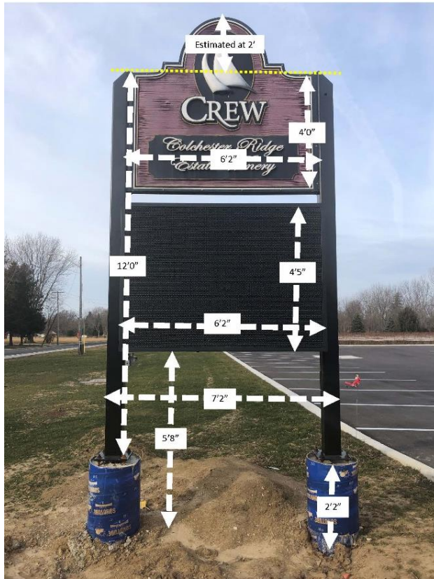
Figure 2. Dimensions of new sign structure as submitted by Town of Essex Building Division
