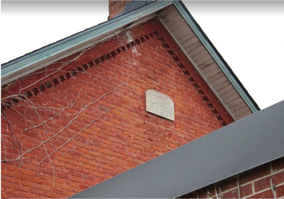
Figure 2. Inset date stone under dogtooth stringcourse brick trim along roofline (Photo Courtesy: Jeremy Parsons, 2020)
