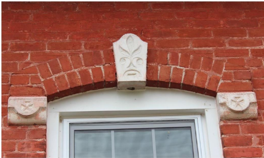
Figure 3. Window voussoir with central keystone carved with floral motif and flanking label stop stones with cross motifs (Photo Courtesy: Jeremy Parsons, 2020)
