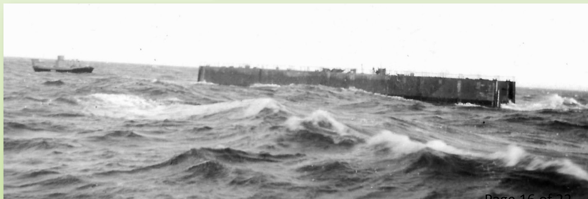
Below: A Phoenix Cassion being towed across the English Channel to Normandy. From the collection of Harry A. J. Brian, RCNVR, Courtesy of David Brian www.forposterityssake.ca .
