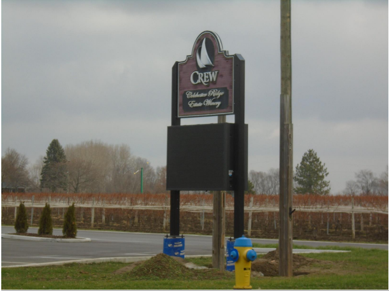
Figure 1. New sign structure with steel posts, logo and electronic media component
